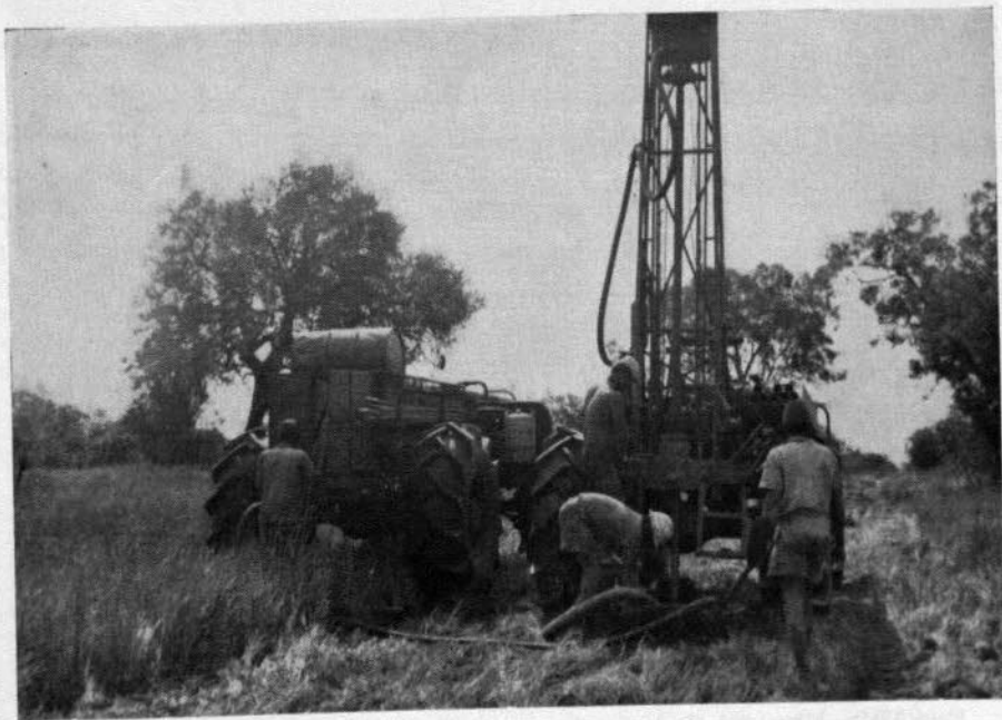
Plate VIIIb—Oil exploration—drilling a shot-hole for seismic prospecting, Coast Province [Photo: J. S. Buchanan, BP-Shell]
