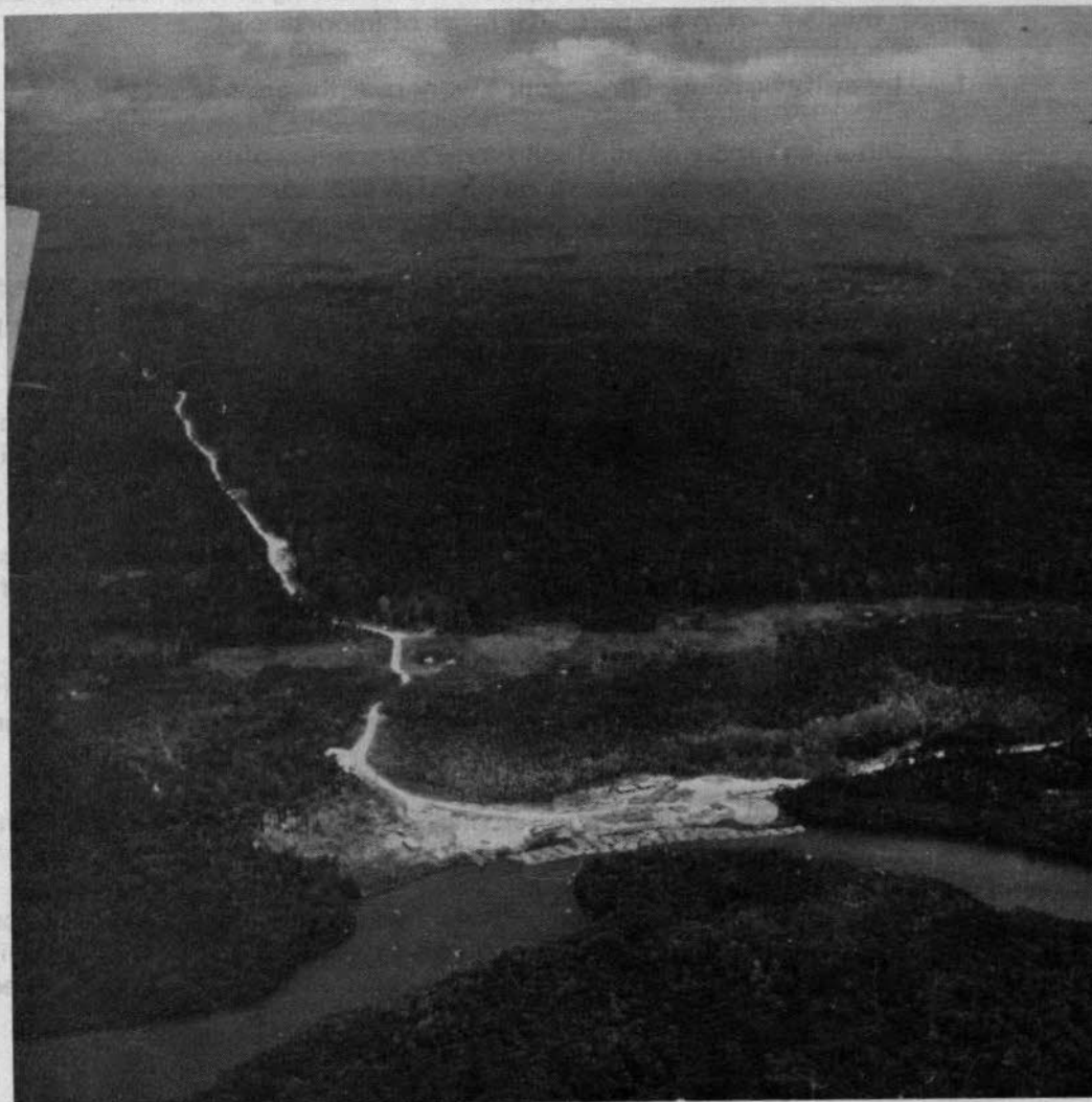
PLATE 1.13 The Dent Hills have a considerable agricultural and forestry potential. Logging road running west from the tip of the Dent Peninsula at Tegupi
