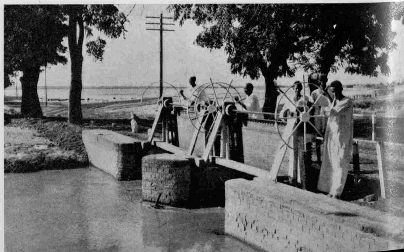
Photo 6. A water control point
