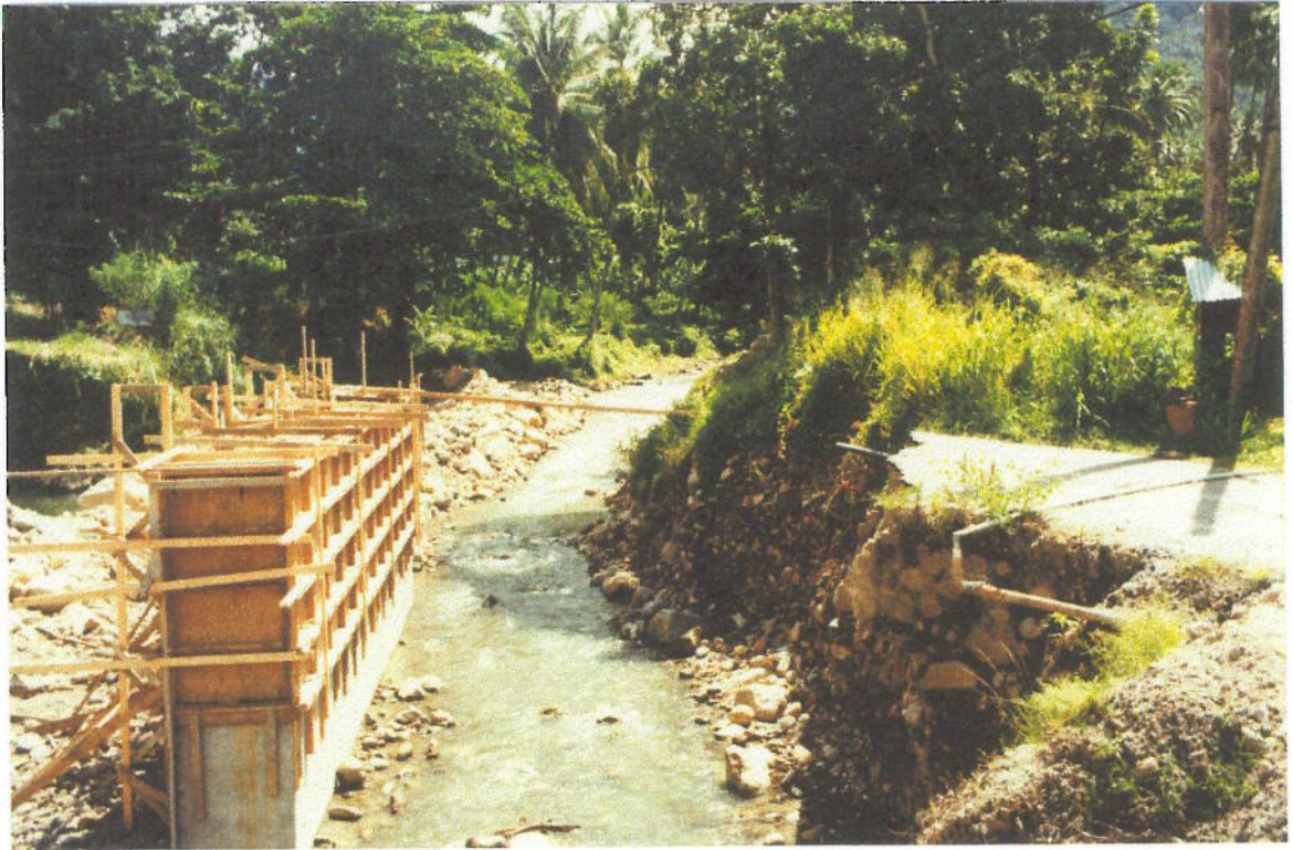
Photo 1 Phase 1 Works: Soufriere Bridge under construction. Looking upstream before 26th Oct.
