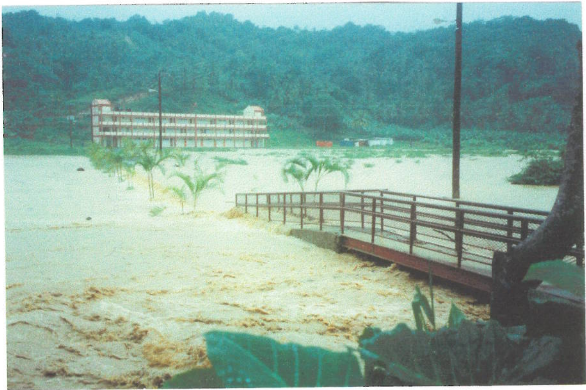
Photo 34 Cul de Sac River : As Photo 33. Oct. 26th. Undercapacity footbridge, floodplain zone.
