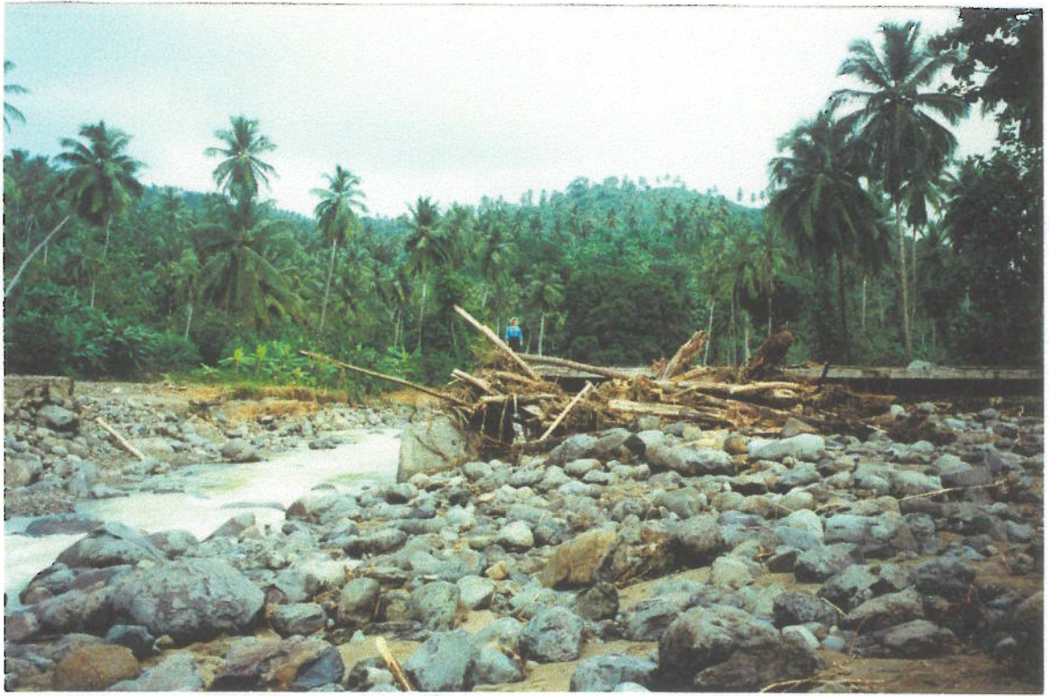
Photo 35 Troumassee River at Mahaut: After 26th October. Bridge blocked by debris then stones.
