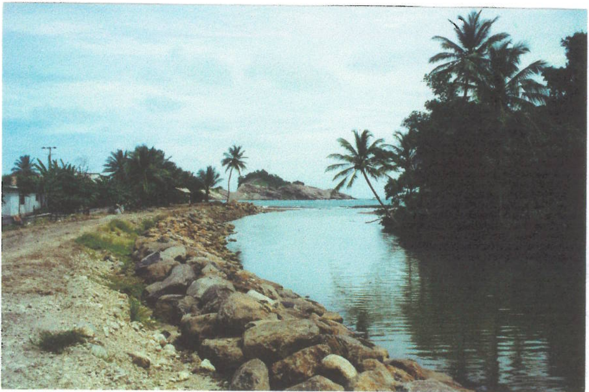
Photo 16 Phase 1 Works: Dennery Town Protection under construction, October 1996.
