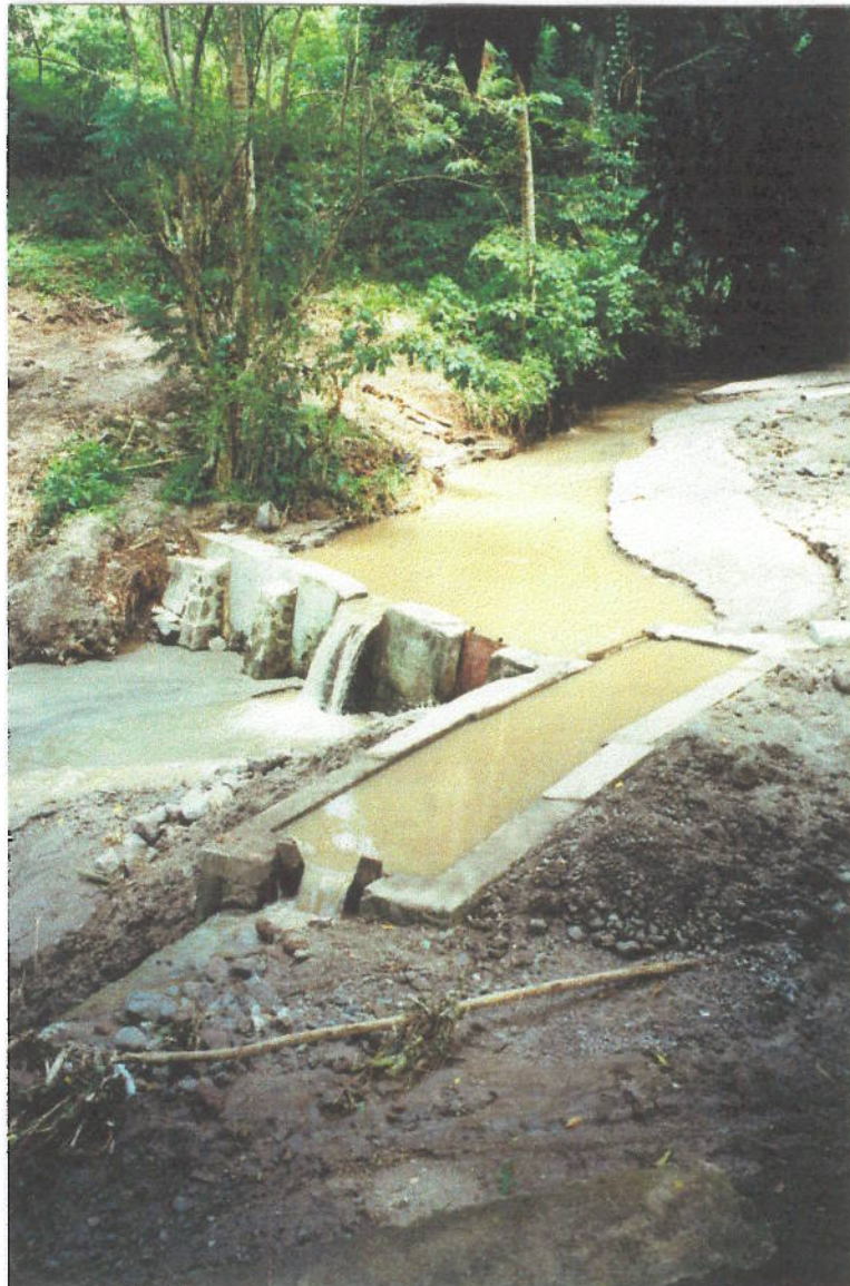
Photo 28 L'Ivrogne River (near Delcer, SW of Island). WASA intake and primary sedimentation.
