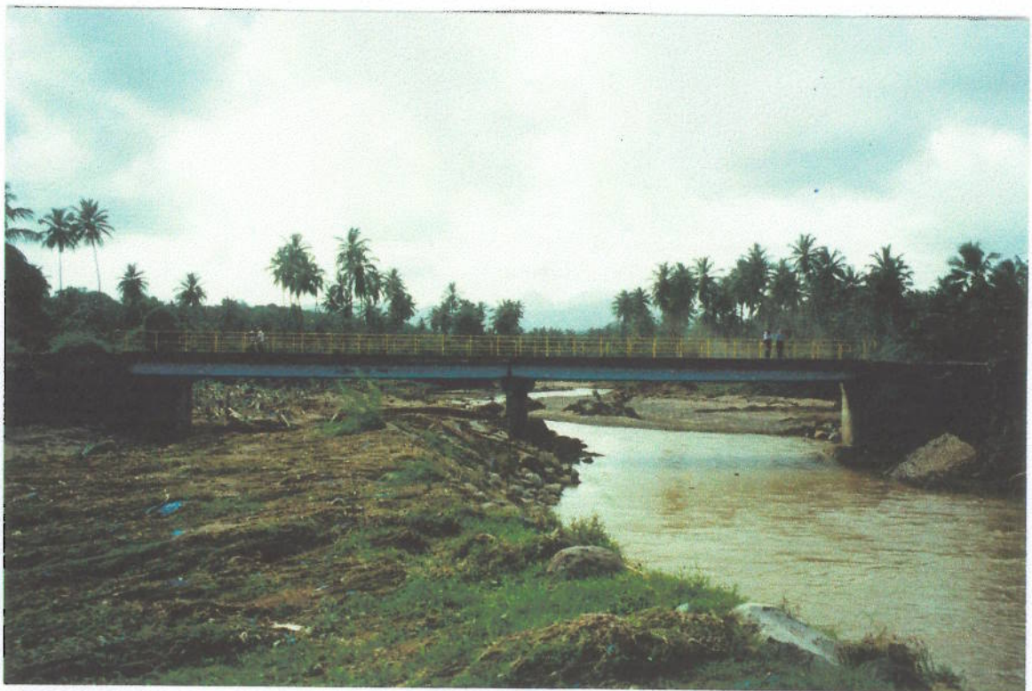
Photo 18 Phase 1 Works: Troumassee Bridge from downstream after 26th- central training works.
